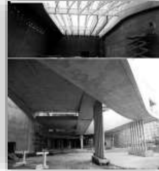
(Figure 3.19) MAXXI Structure Construction
