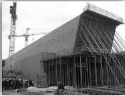
(Figure 3.18) MAXXI During Construction
