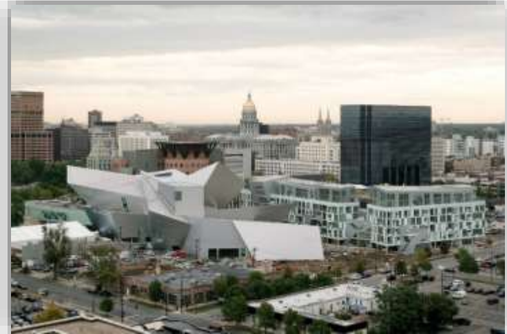
(Figure 3.31) DENVER Art Museum – General View
