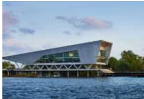
Water institute headquarter
