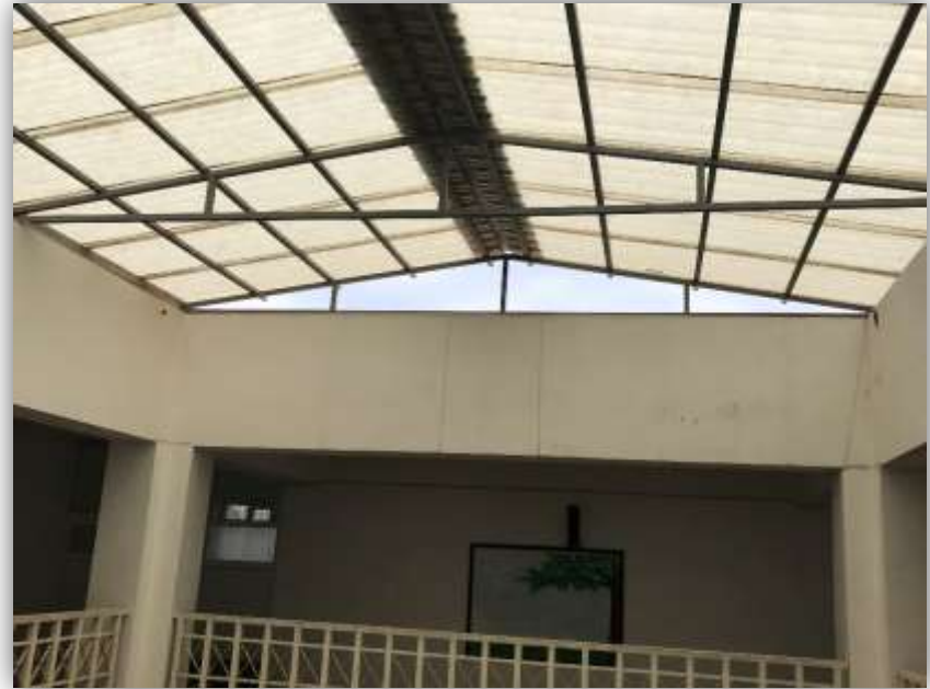
Court Working as Skylight
