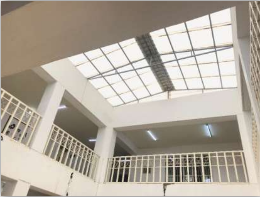
Court Working as Skylight
