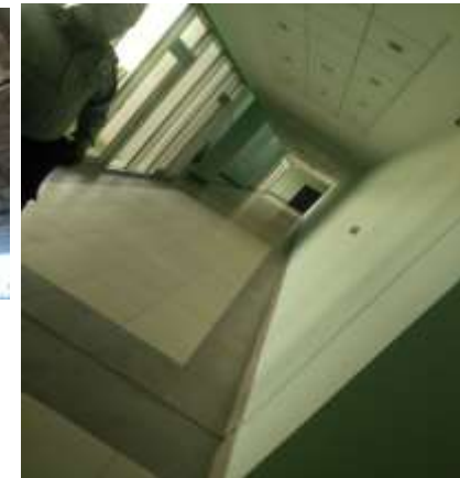
For wall used(block,morter,chipsem cement,paint)
